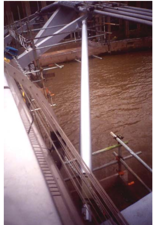
FIGURE 8 PIER DAMPERS
