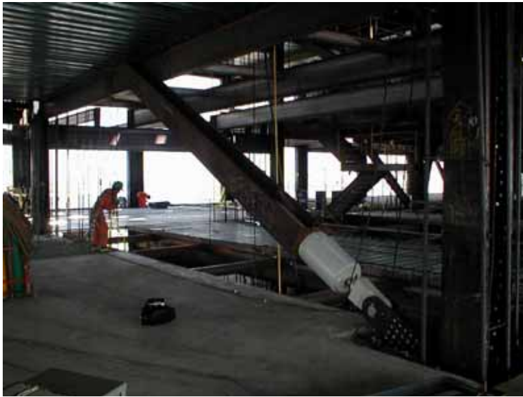
FIGURE 13 DAMPER INSTALLATION
