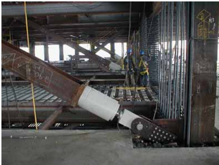
FIGURE 12 DAMPER INSTALLATION
