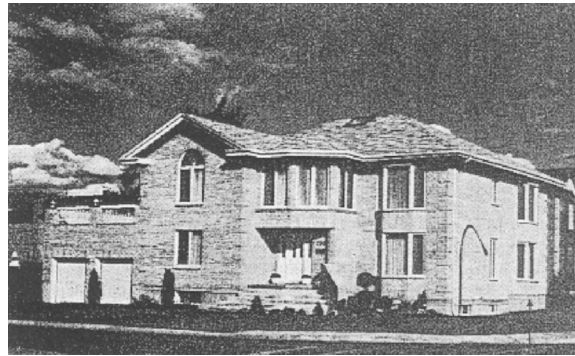
Figure 5. Photograph of wood-framed house with sliding base isolation system. (From Pall and Pall 1991, © University of Toronto Press. Reproduced with permission.)
