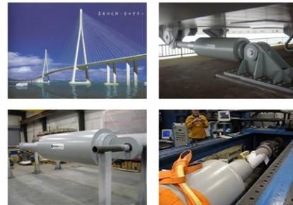
Fig.4 Sutong Bridge and dampers
