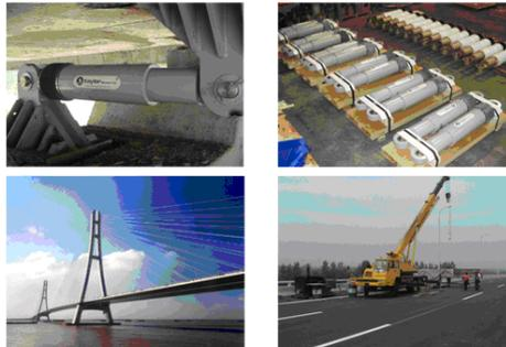
Fig. 1 Nanjing Yangtze river 3<sup>rd</sup> bridge and 54 dampers
